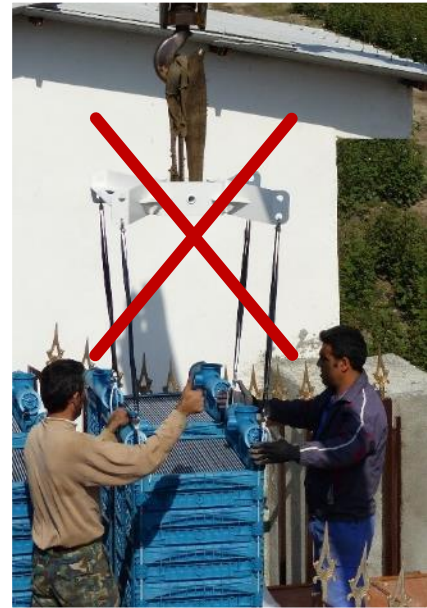
Figure 26: Lifting a tower with the Lifting Tool. The coil-loops must be exact vertical
