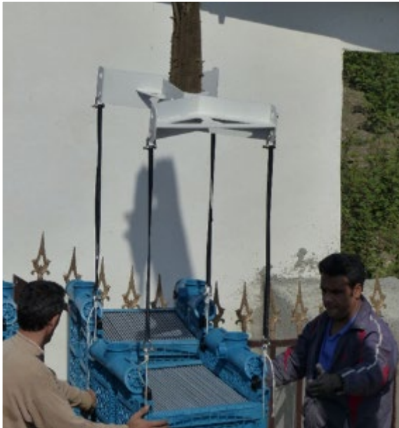
Figure 26: Lifting a tower with the Lifting Tool. The coil-loops must be exact vertical
